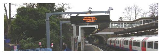
The Free Standing Gantries are designed to suspend VEID Units safely on open platforms. They should be securely mounted to new concrete foundations.
